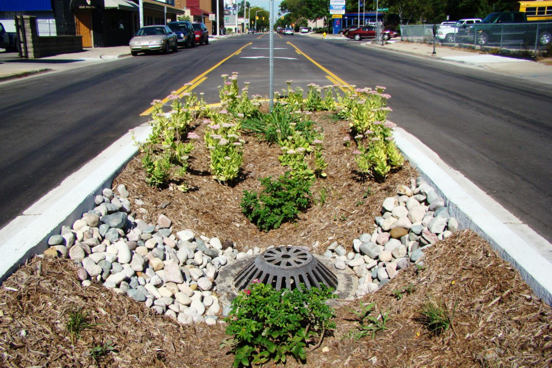
Grand Rapids Plainfield Avenue Bio-retention Basins
